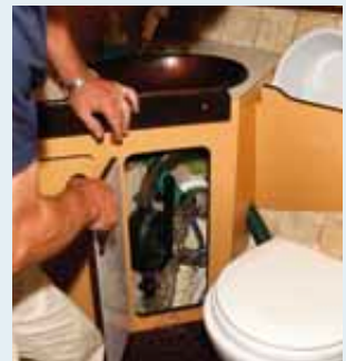
Access to seacocks can be bad so expect to work one-handed
