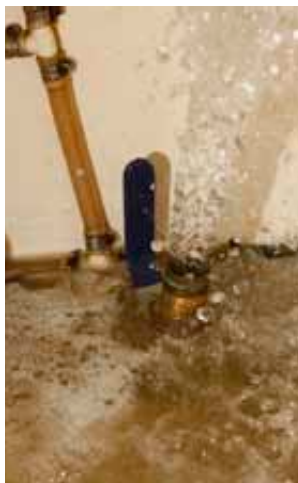
ABOVE: We removed the galley sink drain pipe and opened the seacock to create a gusher
