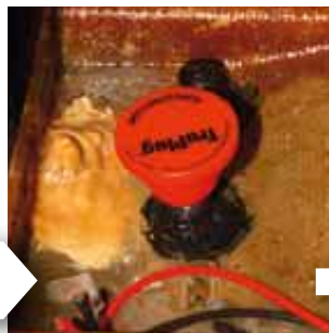
With a damaged log pipe, the TruPlug formed a perfect seal and stopped the leak completely
