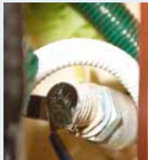
The cracked toilet outlet tailpipe left an irregular hole to block
